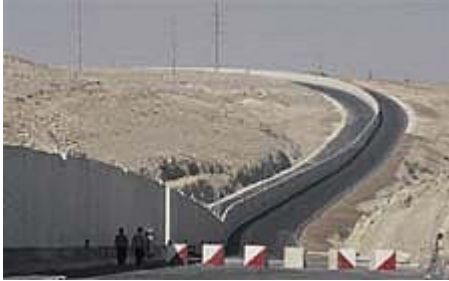
A completed section of the security barrier near Ma'aleh Adumim.
